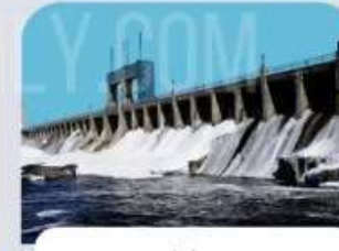
Dam Holding Water
