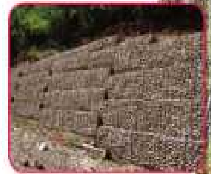
This rock wall will keep soil from moving down this hillside.
